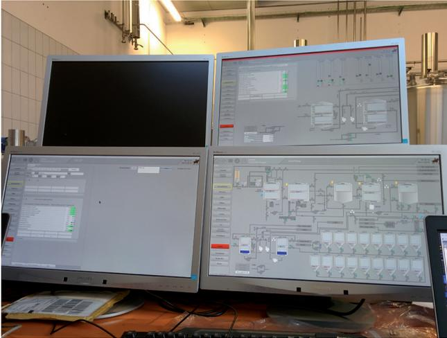
*The Master Brewer can keep track of the entire production process at a glance on the multiple monitors displaying supervision application information in the control room.*
