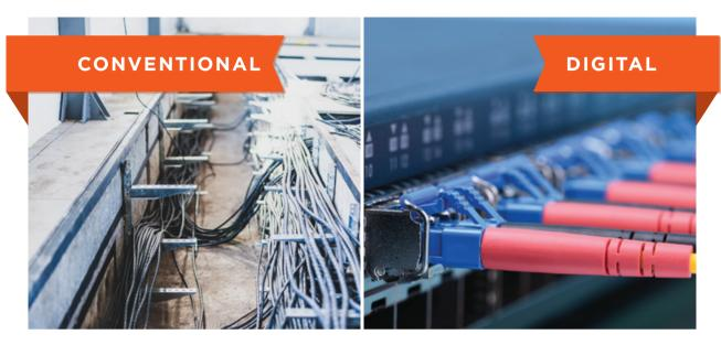
IEC 61850 enables complex cabling to be replaced by network or fiber optic cables and thus promotes flexible but secure signal transmission instead of rigid wiring of signals to safety equipment.
