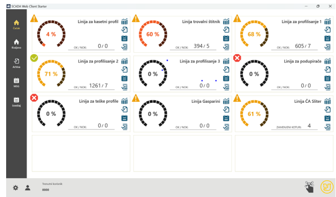
Main screen (dashboard) for all lines at the Čačak site
